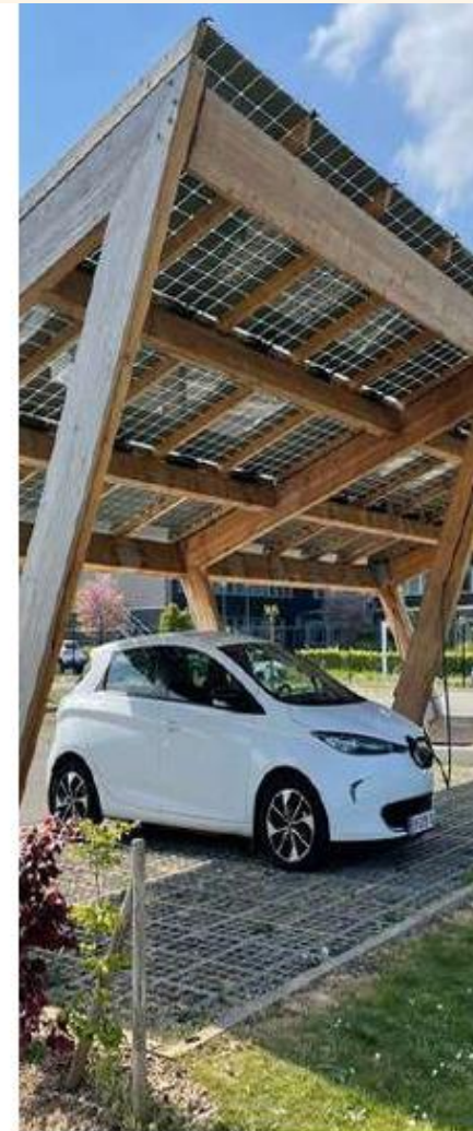
Ombrière © Rossini Energy
